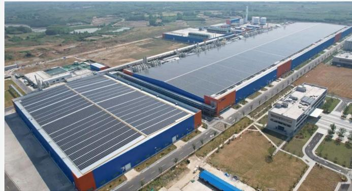
Here is a photo of the 19.8MW BIPV project at Chuzhou EGING Base
